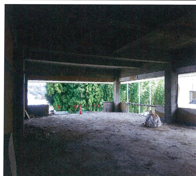
NO. 7 2F大会議室内装解体0818 2015-08-18
