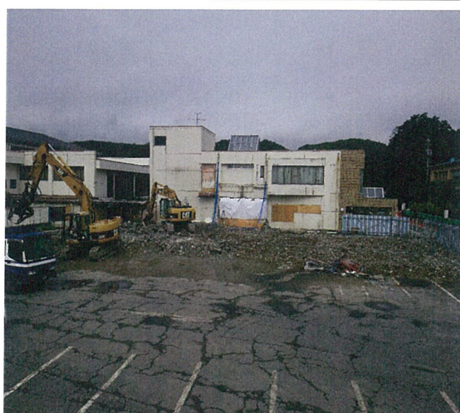
NO. 11 上屋・土間躯体解体完了0907 2015-09-07
